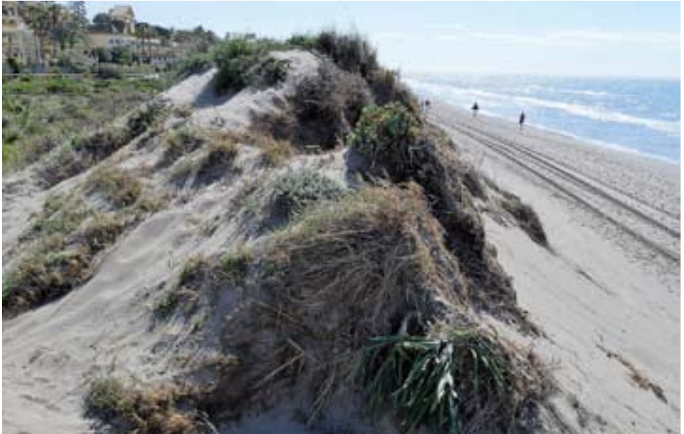
5.7.7 View of the embankment at the far western end.
