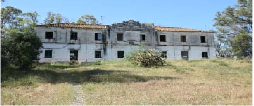
4.3 Headquarter of the Guardia Civil in Real de Zaragoza
