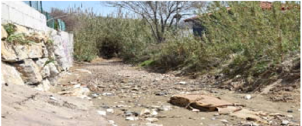
2.8 View of the mouth of the Sequillo stream, invaded by constructions and reed beds.
