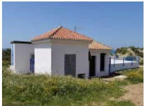
4.4 Sewage pumping station.
